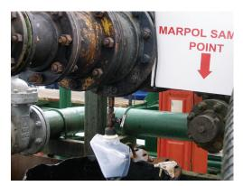
Fuel oil sampling is an essential element of any bunkering operation.
